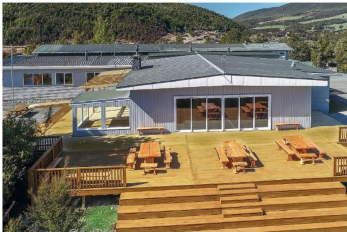
The newly refurbished Rotoiti Lodge.
